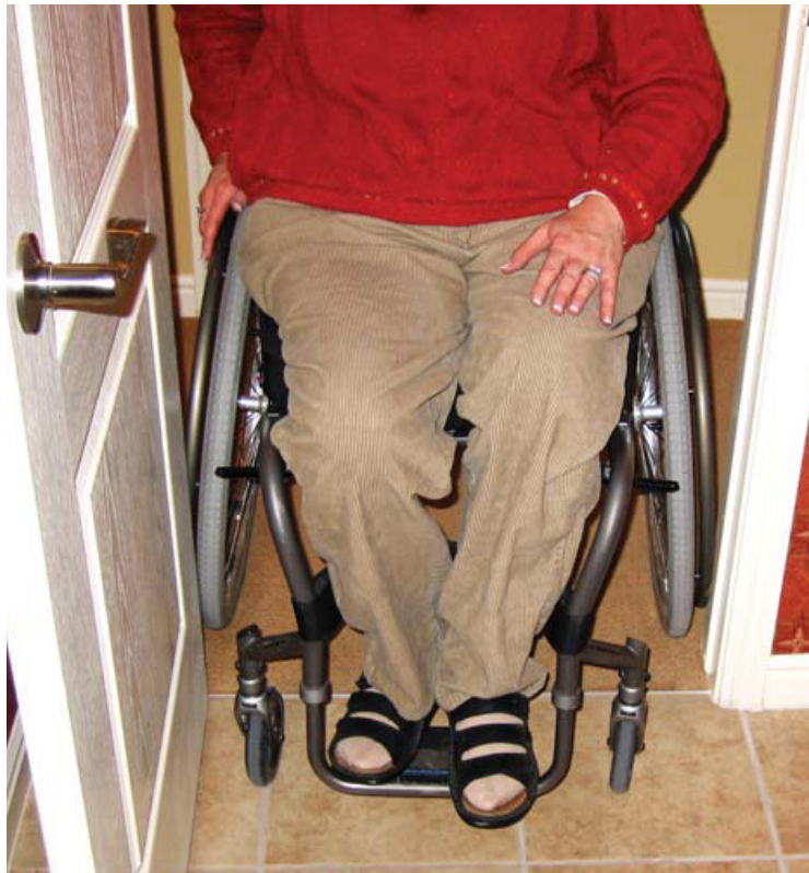
28 inch wide bathroom door
