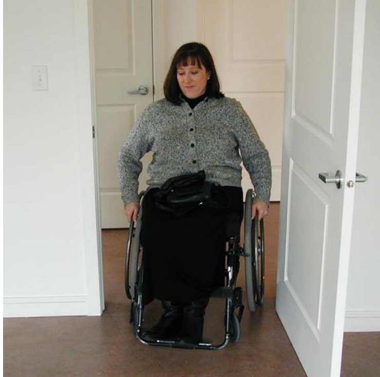
36 inch wide interior door
